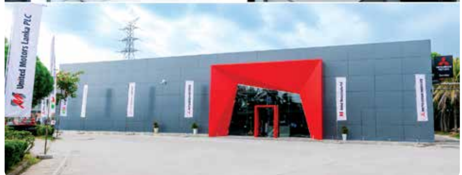
New service reception and customer lobby at the Orugodawatte main workshop
